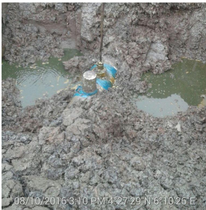
Fig B: Incident facility after excavation/Spilled Crude Oil
